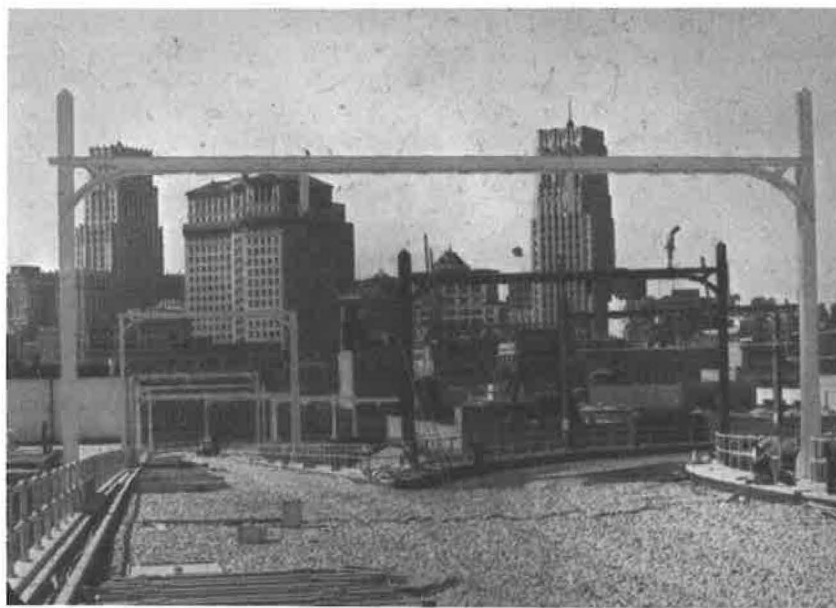
FIGURE 6 Terminal viaduct under construction. Note gravel track ballast and overhead trolley wire support frame. Trains proceeded counterclockwise at the gore. Source: Caltrans.
