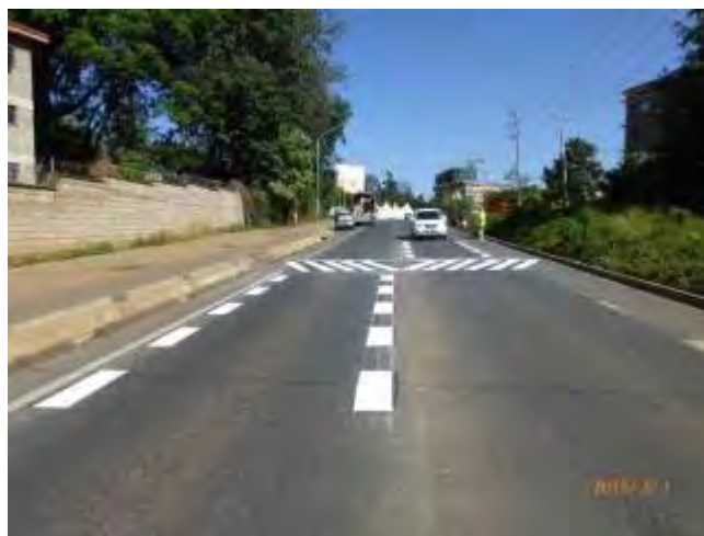
Clear lane markings warn motorists of the hump. This is particularly helpful at night.
