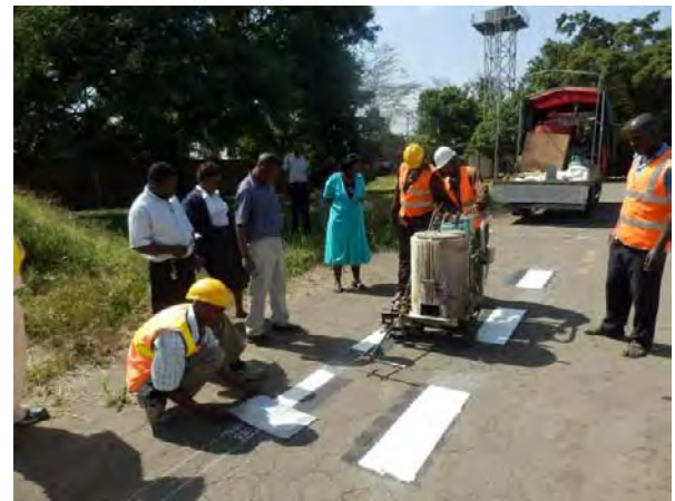
Test construction in MTRD yard and observation by MTRD engineers. (2015.1.27)
