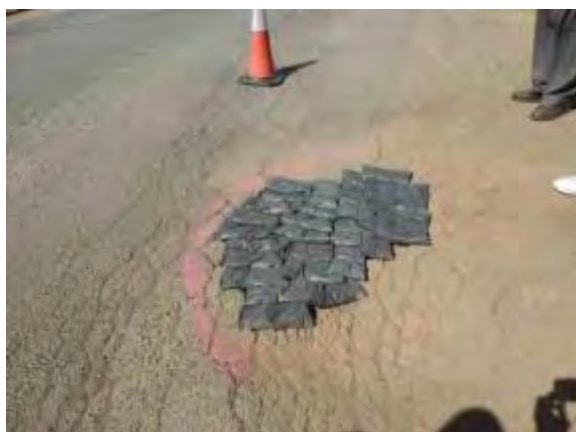
Included in the MPP is an effective method of repairing potholes using special patching materials
