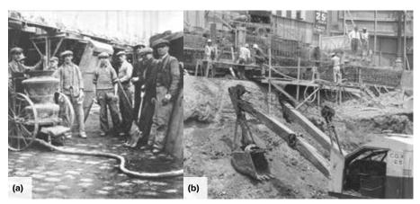
Shotcrete has been widely used for over a century: (a) a crew poses with their equipment in the 1920s; and (b) a crew places a foundation wall in the 1940s
