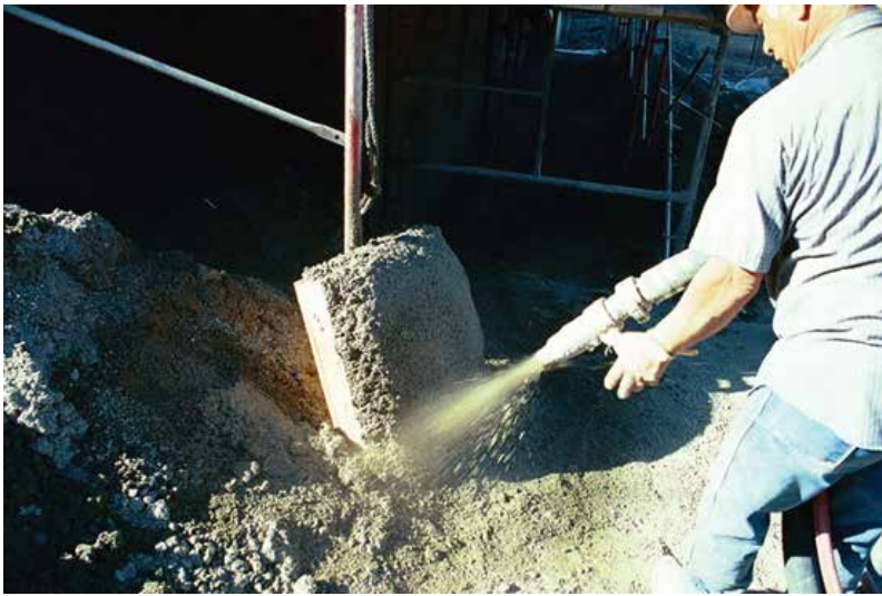
Fig. 4: A typical shotcrete test panel being shot during construction
