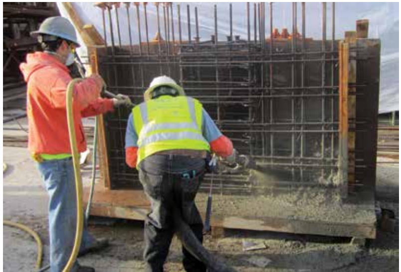
Fig. 1: A typical preconstruction test panel with congested reinforcement
