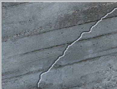
Structural Crack and Void Repair
