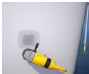
Chamfering of damaged area.
