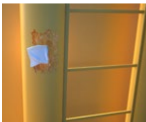
Cleaning of damaged surface.
