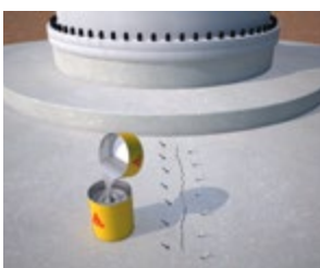
Mix the Sika® Injection-458 pre-batched A+B containers.
