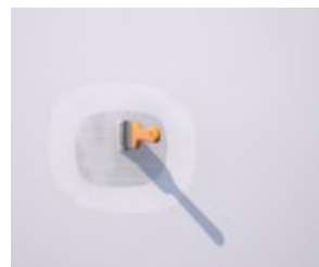
Application of fibre patch and adding Sikadur® Blade Repair Resin.
