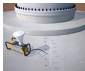
Apply the epoxy resin using a 1-component injection pump.
