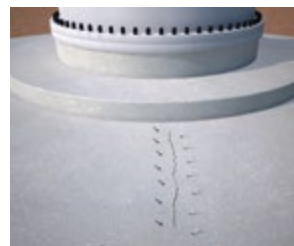
Insert the injection packers.
