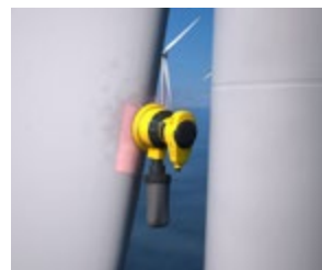
Sanding of repaired area.
