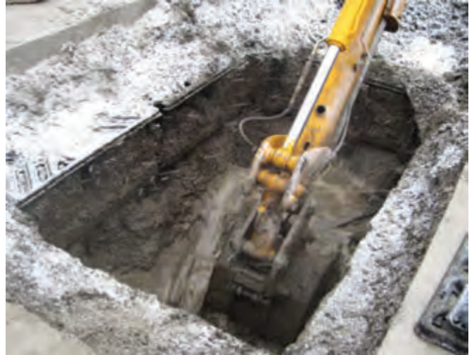
Excavation below bottom of soil cells to daylight water pipe.
