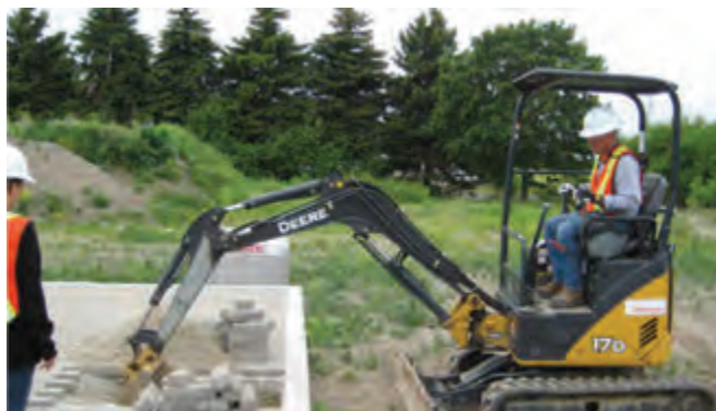
Removal of pavers and granular base.
