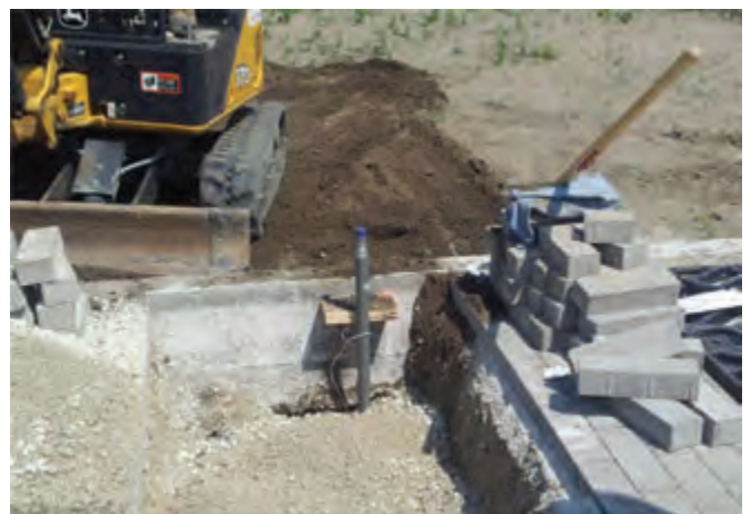
Backfill and ensure riser is set correctly. Conclusions of the Enbridge Gas exercise
