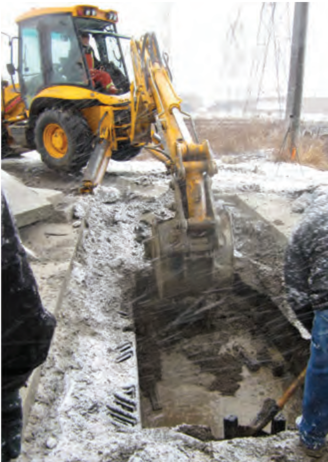
Mechanical removal of soil cells.
