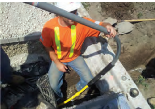
Riser is attached and pulled through.
