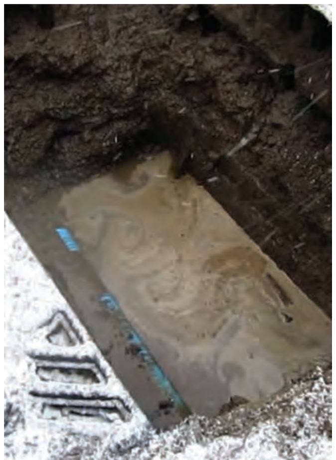
Excavation below bottom of soil cells to daylight water pipe.
