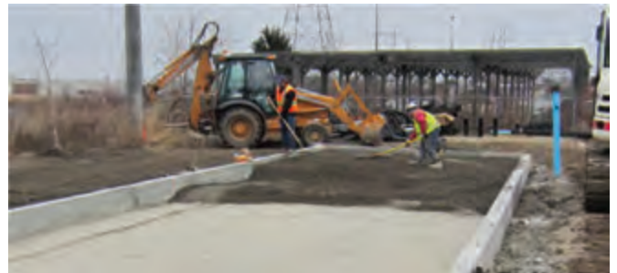
Backfill installation on top of deck.
