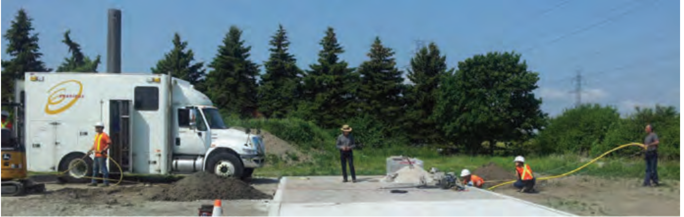
Pulling the lateral through the cells and growing medium.
