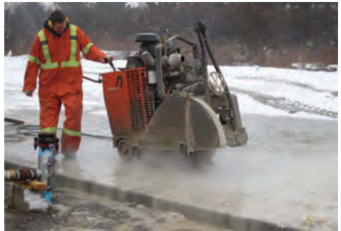
Sawcutting concrete pavement.
