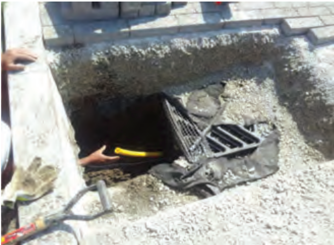
End of lateral at building end.
