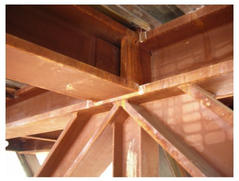
Photo 9: Typical full penetration welded connection of the bridge truss structure.
