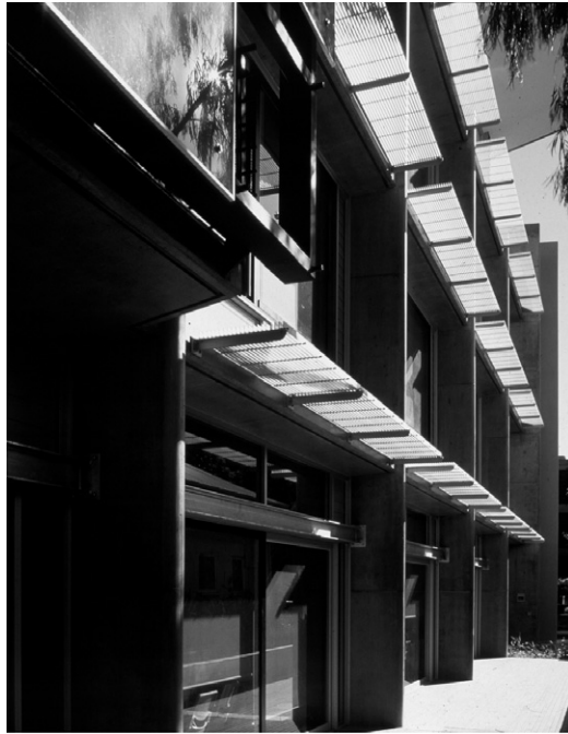
Figure 27.6 Horizontal sunshades on the northern façade.
