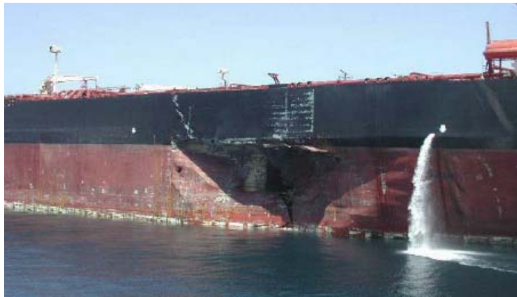
Figure 5-2: Side structure damage of a tanker resulting from a collision (Wang et al 2003).
