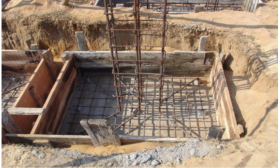
Figure 2.7: Column footing
