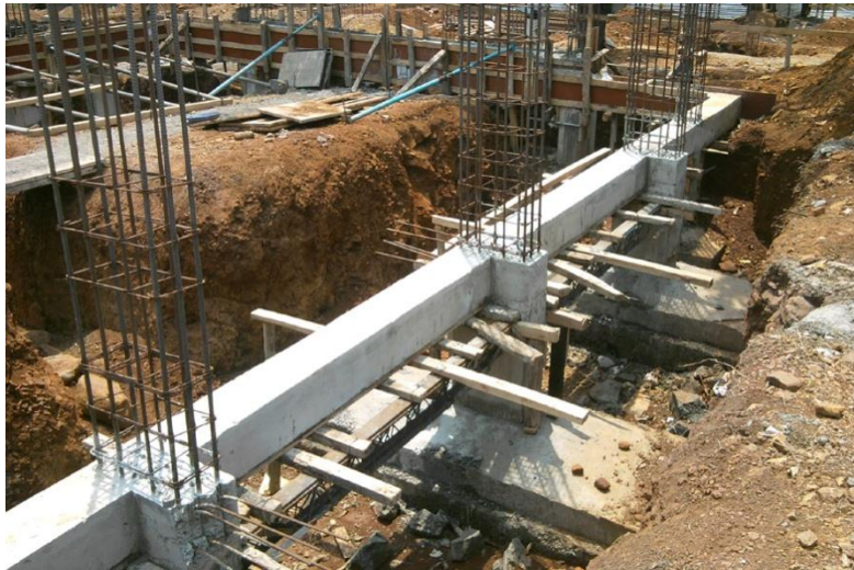
Figure 2.9: Strap footing
