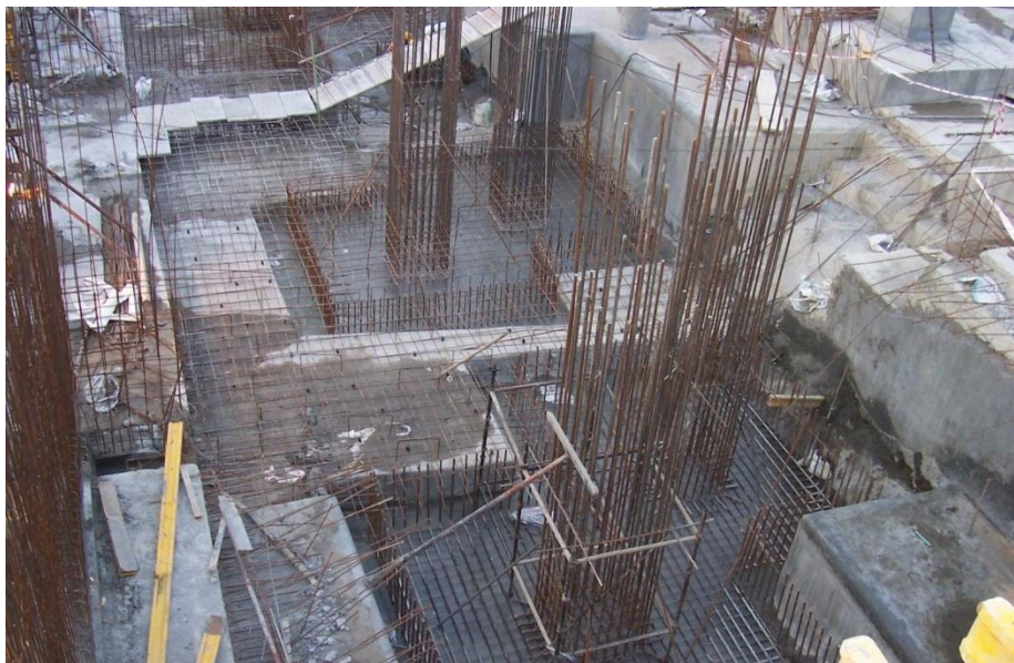
Figure 2.8: Combined footing
