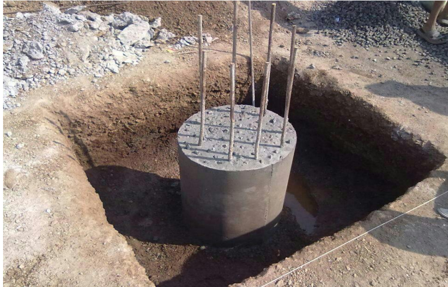
Figure 2.11: Pile foundation
