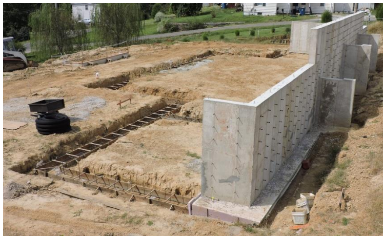
Figure 2.6: Wall footing
