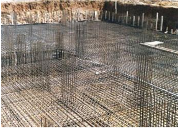
Figure 2.10: Mat or raft foundation
