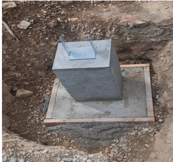
Figure 2.12: Pier foundation
