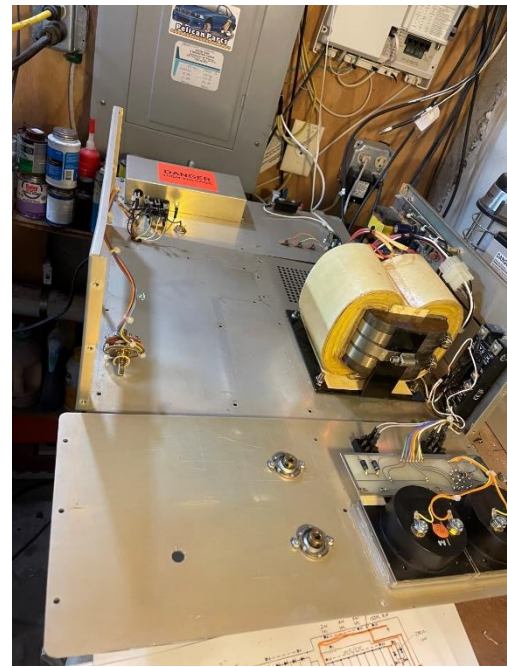
The front and the rear panels have been removed. The RF deck also has been removed.
