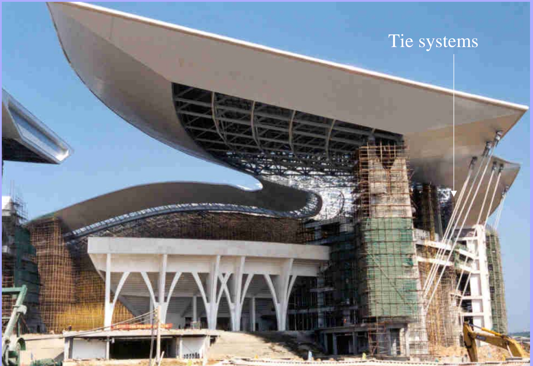
Tie systems to stabilize the cantilevered roof
