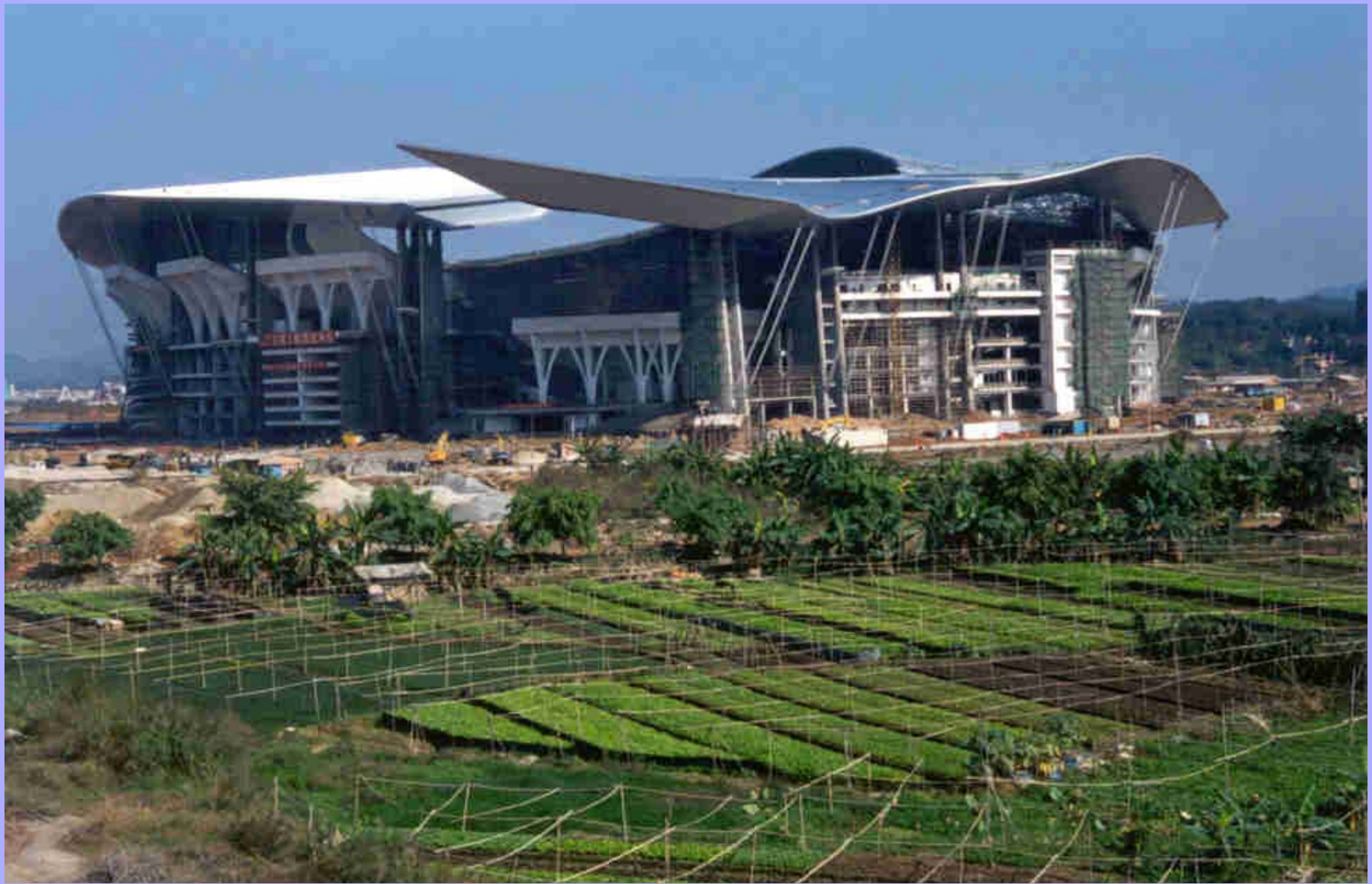
External view of Stadium
