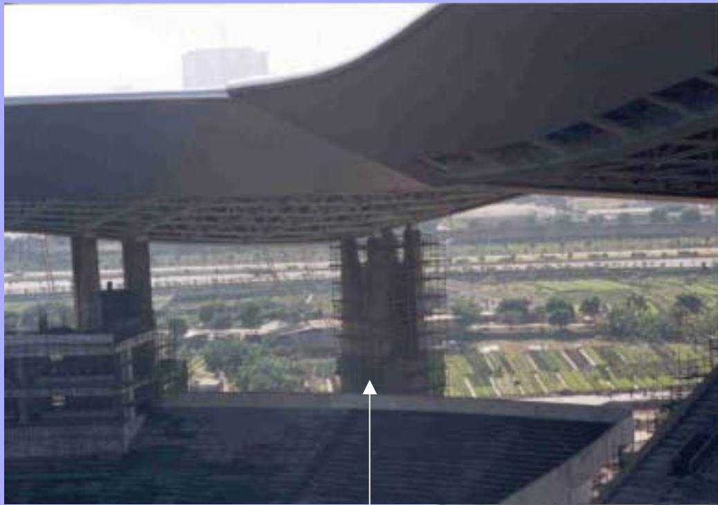
Piers supporting the cantilever roof truss
