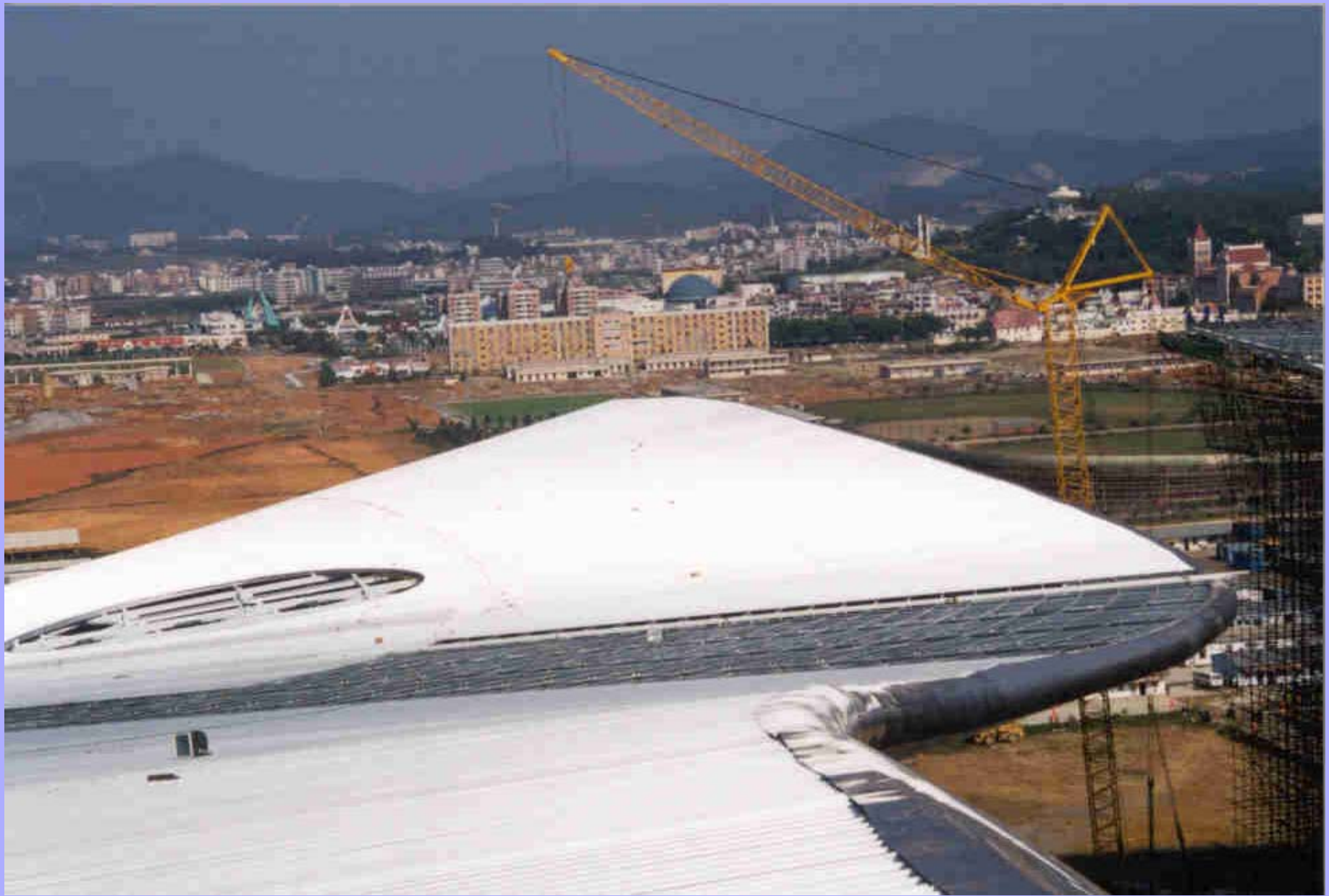
Decking system of the roof
