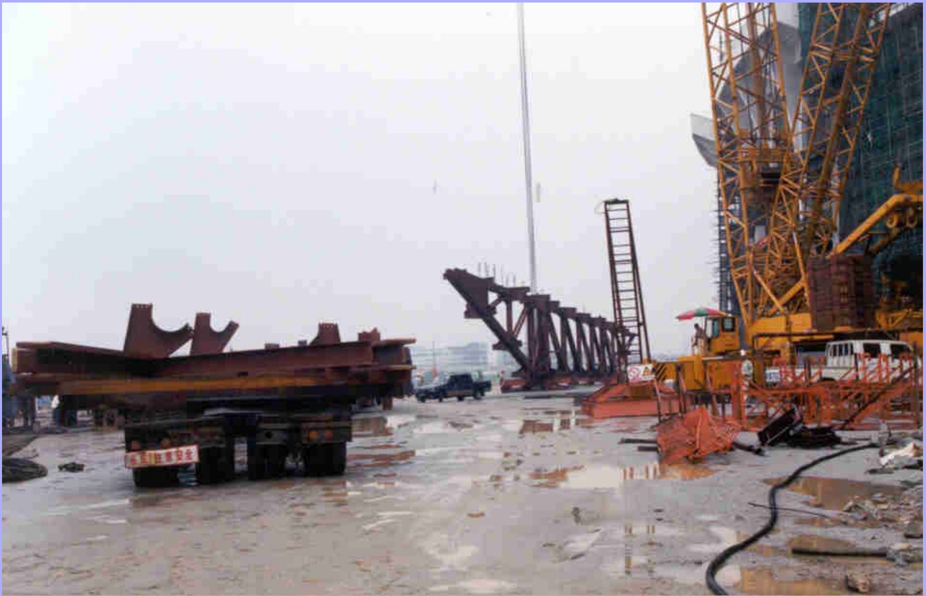
Hoisting the cantilever truss
