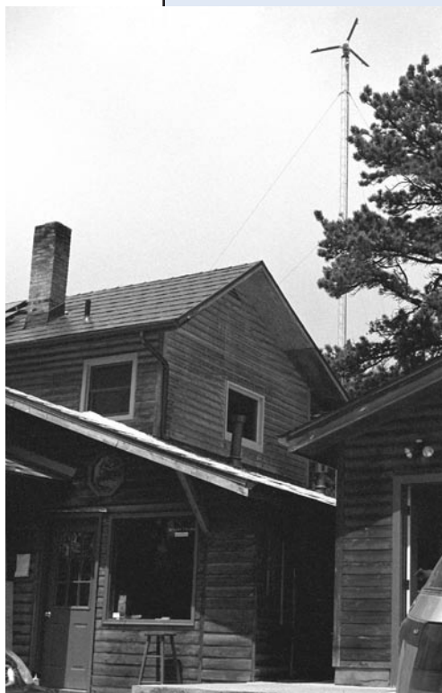
Jim Green, NREL / FTX02796
