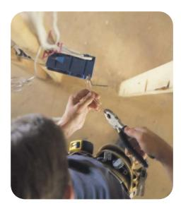
For an additional fee, you can hire AT&T or an electrician to complete the inside wiring
