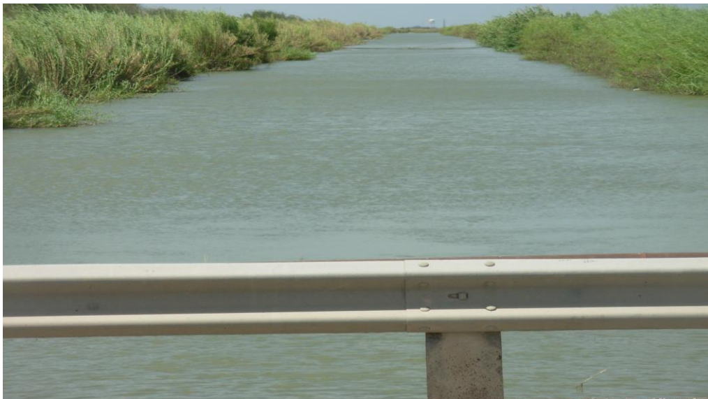
PORTION OF DONNA MAIN CANAL (Looking North Towards Donna, Texas, From Highway 281 Bridge, 08/05/11)
