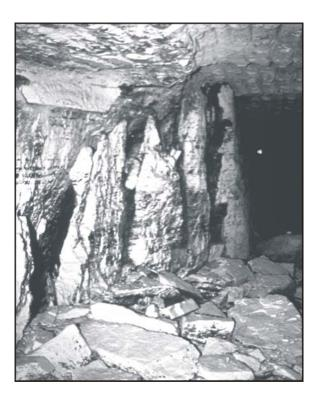
Figure 3.—Skin failure of unsupported rib.
