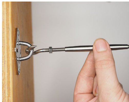
Fig 6.1 Tension the cable by tightening the turnbuckles at each end. Hand Tighten ONLY !
