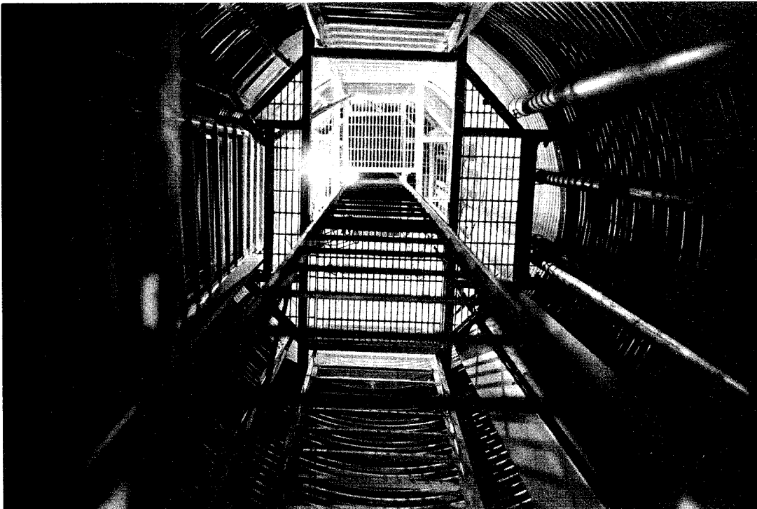
Looking up the utility shaft at Region 8.
