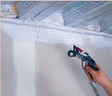
The Head-of-wall construction joint is sprayed with the fire resistive sealant.
