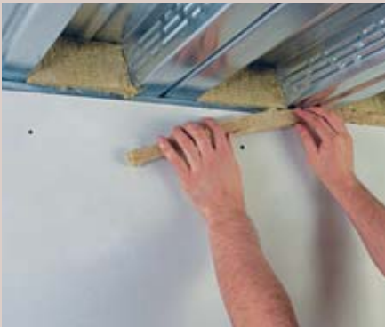
The deflection gap is filled with Mineral Wool.
