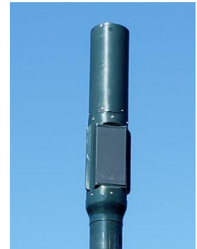
Example shrouding for uncovered panels.
