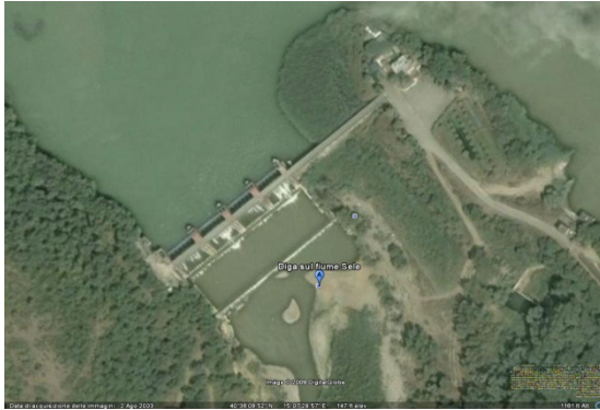
Figure 3: Aerial image of the dam.
