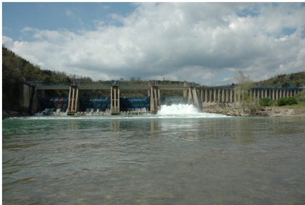
Figure 4: Frontal view of the dam.
