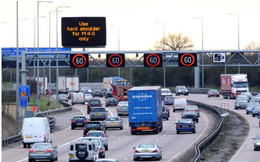
Figure 1 - Dynamic hard shoulder running - to be brought to an end
