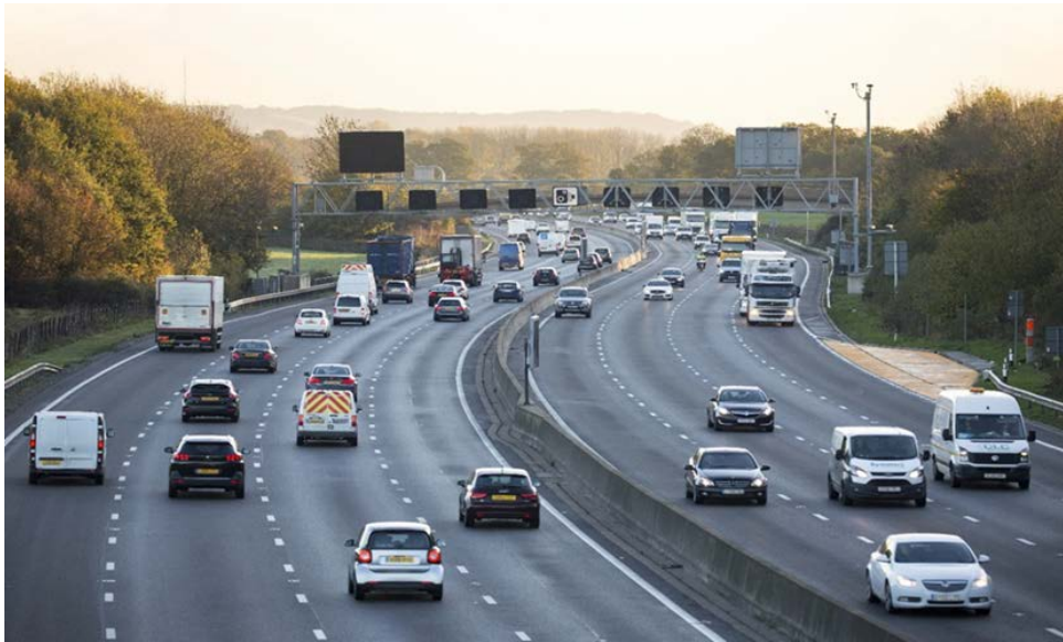
Figure 2 - All lane running smart motorway
