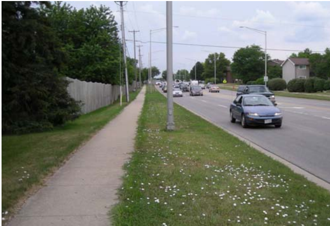
This 9 foot buffer provides good separation for pedestrians from motorists. Wide buffers are especially desirable on roadways posted at 35 mph or higher.
