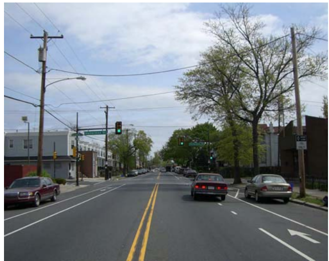
Torresdale Avenue in Philadelphia, which functions as a community collector in an urban area, has 11 ft. travel lanes, 5 ft. bike lanes, 8 ft. parking lanes, and 6 ft. sidewalks.
