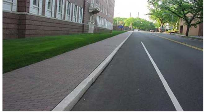
Rutgers University in New Brunswick, NJ striped a shoulder on George Street through its central campus as the most expedient way to create a facility for bicyclists.
