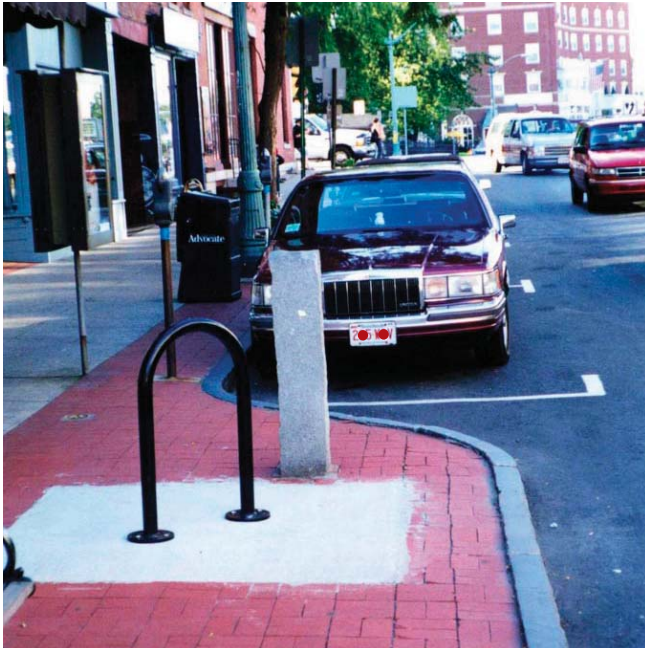
In addition to improving sight distance of and by pedestrians, a curb extension provides room for a bike rack in a constrained urban area.
