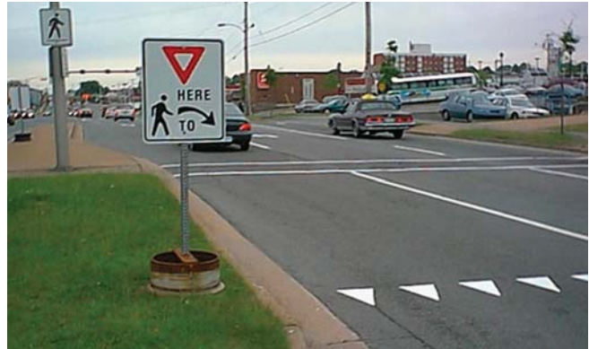
Advanced yield markings are recommended in conjunction with uncontrolled pedestrian crossings on multi-lane roadways to reduce the possibility of multiple threat crashes.
