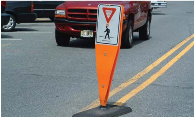
Yield to pedestrian signs mounted on the centerline of two-lane roadways have proven effective in increasing the yielding rate of motorists, and are highly recommended for urban areas.
