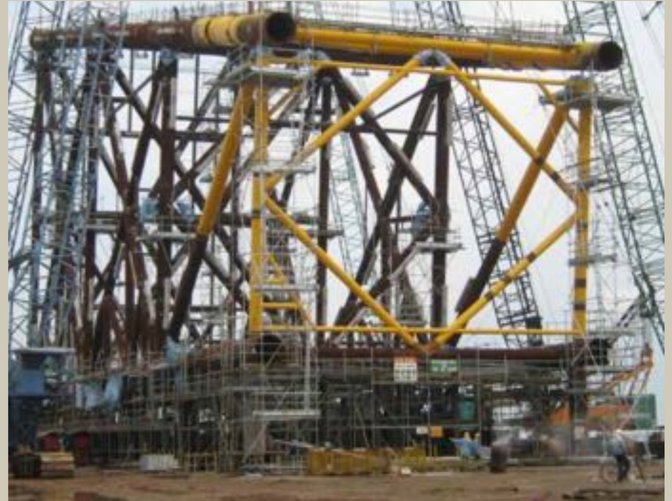
Vasai East Development Project – Jacket Top Panel Erection
