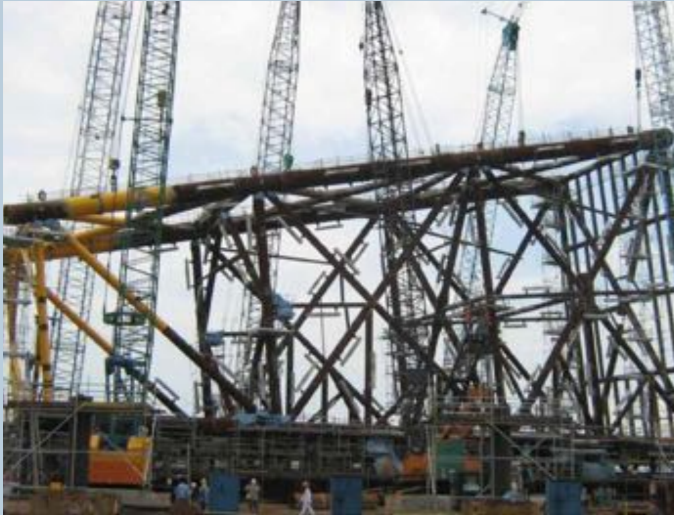
Vasai East Development Project – Jacket Top Panel Erection
