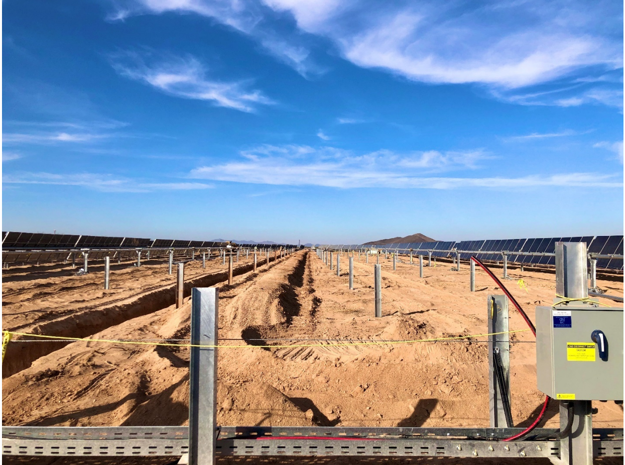
Figure 1 – Driven Post Installation
