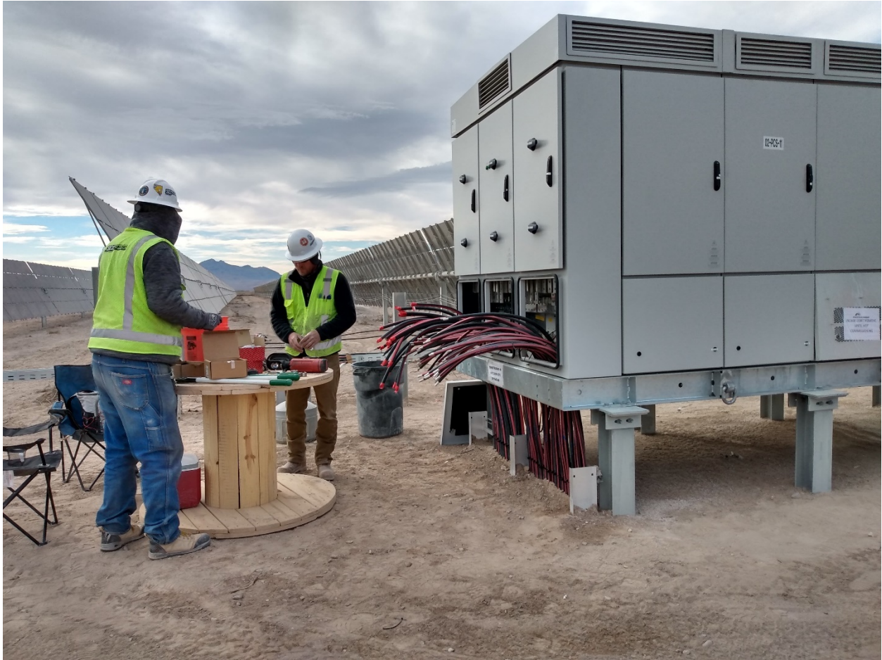
Figure 4 – Solar Inverter
