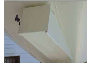
Poke Hole 8" x 8" access to discharge just above gate.
