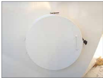
Roof Manhole Access hole in top cone.
