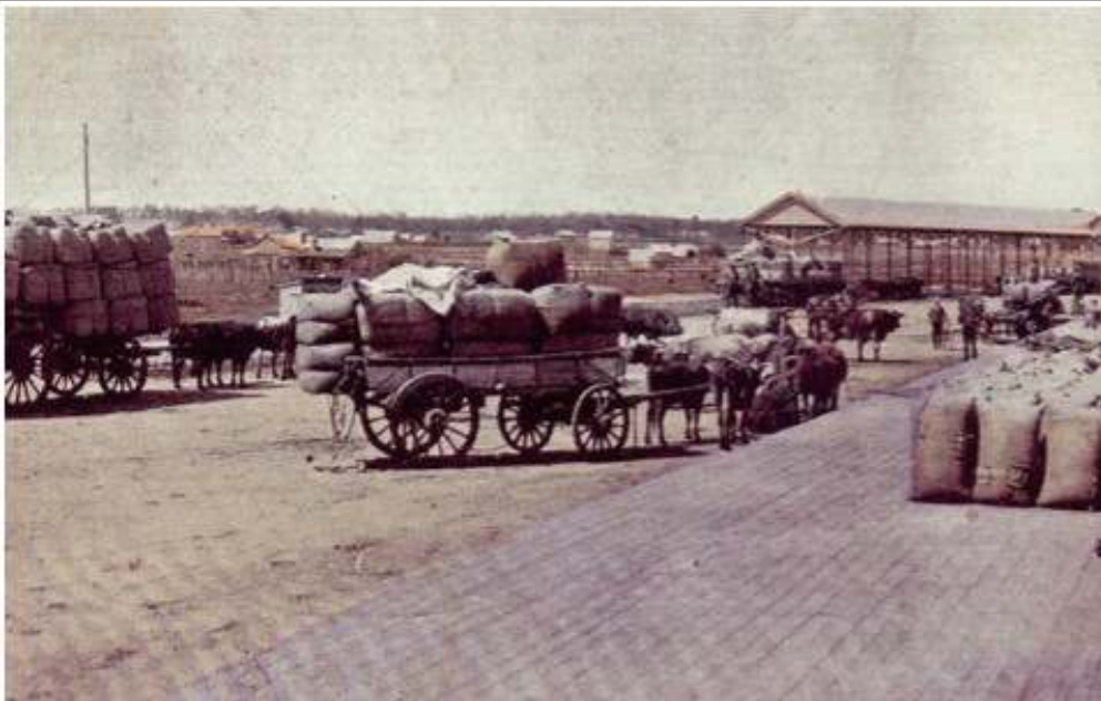
Temora railway yards 1906. View is over landing stage towards Victoria Street.
