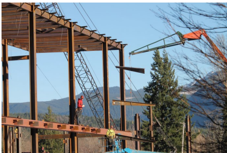
(Photo above) Steel girders are hoisted into position.
