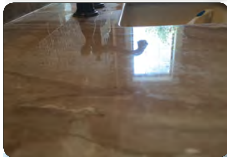
Before and after photos of a vanity restoration. Proper documentation and client testimonials can be key factors in the success of your restoration business.
