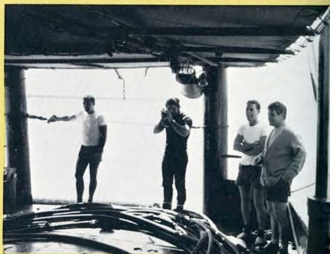
"Taking five" while working on the cable off Portsea, Victoria, these four Party 87 men are (from the left): Maurice Blaize, Lee Warner, Guy Harder, and Gordon McGarry. All are local helpers.
