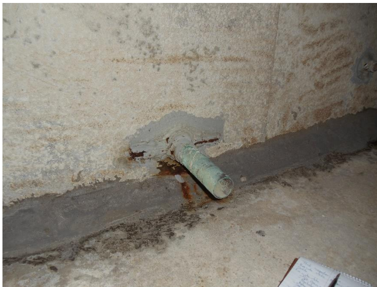
Image 4 - Water level Pipe Penetration
