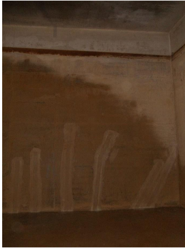
Image 1 - Repaired Cracks
