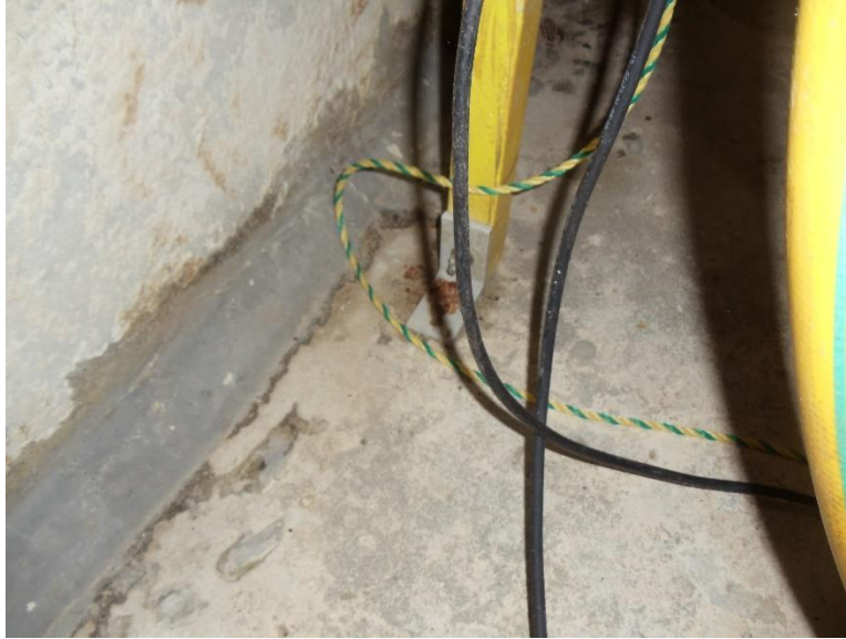
Image 5 - Corroded ladder anchors
