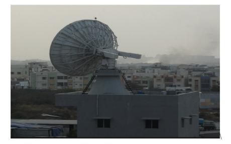
Figure 1: X-Band Polar Satellite Antenna
