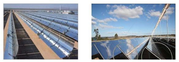
Figure 5. Parabolic trough (left) and linear Fresnel (right) collector systems (photos from <u>http://en.wikipedia.org/wiki/Solar\_thermal\_energy</u>).
