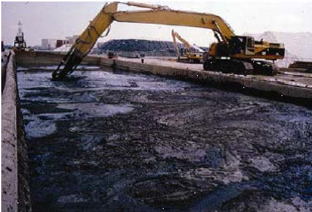
Figure 29: Ex-situ for on-site use stabilization (mixing in place of contaminated dredged materials) (Wiki, unpublished document)
