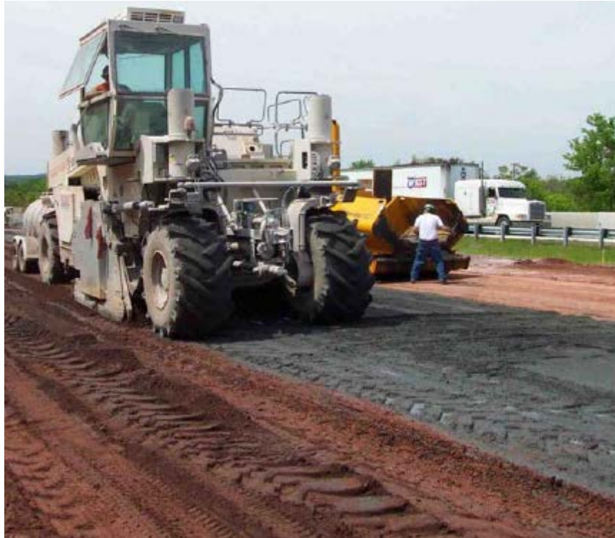
Figure 2: A road reclaimer mixes soil with moist conditioned fly ash (Beeghly, 2003).
