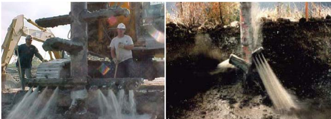
Figure 6: Parts of wet mixing tool showing injection of slurry into the soil (Porbaha et al, 2005)
