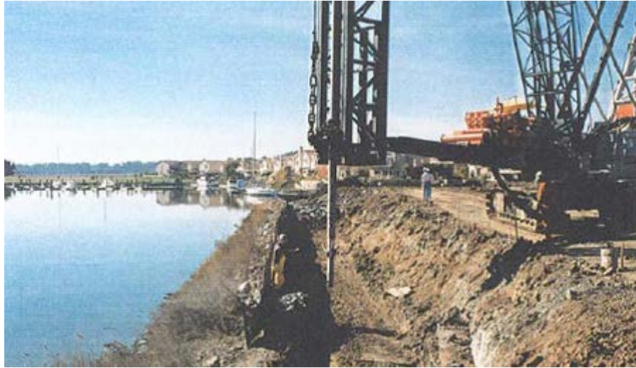
Figure 23: Liquefaction mitigation along river bank at Napa Yatch club, California (Porbaha et al, 1999)
