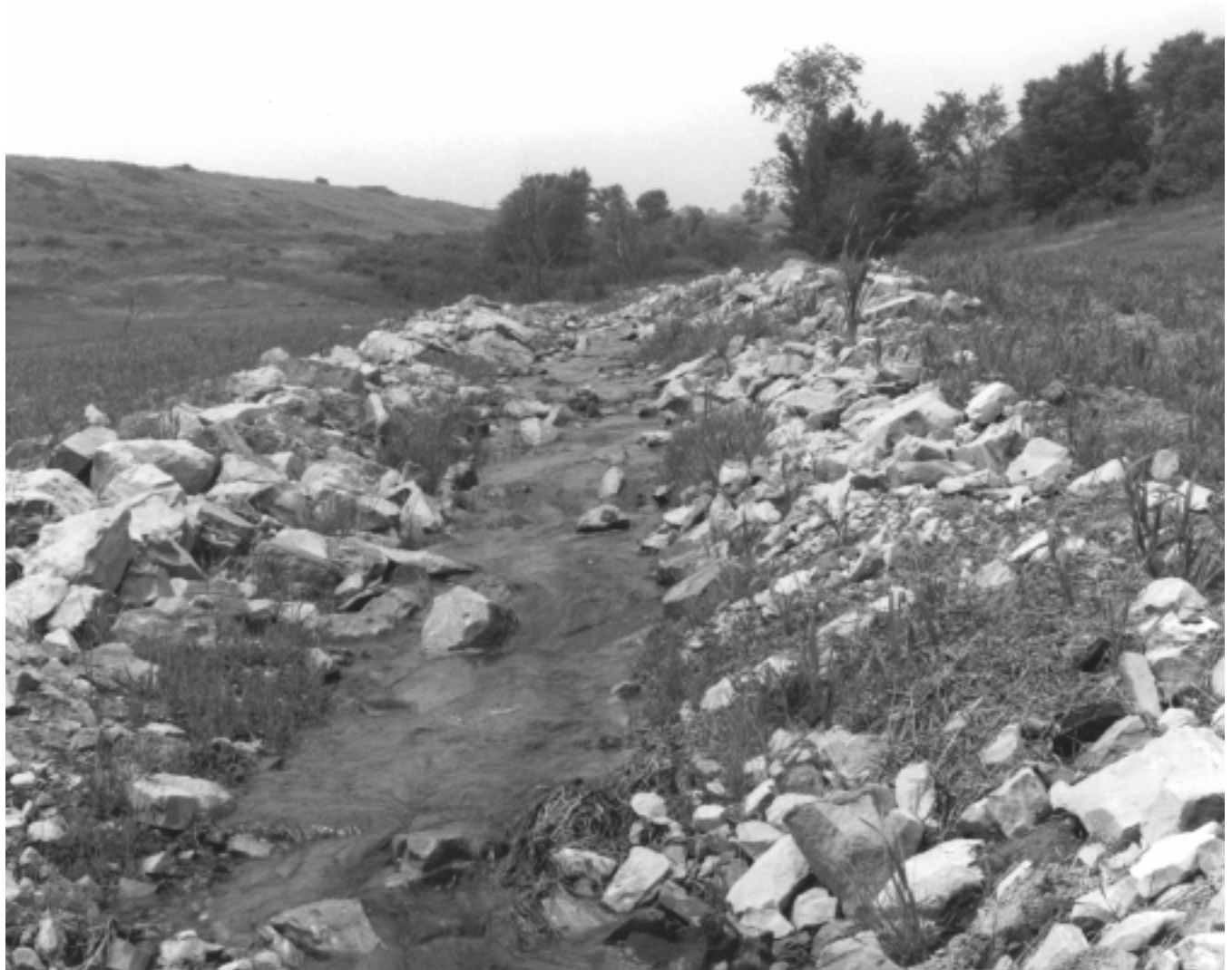
Figure 9.—A drainageway lined with riprap in a reclaimed area of Morristown silty clay loam, 8 to 25 percent slopes.
