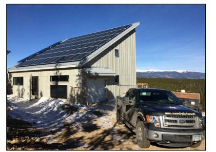
20.52 kW PV, 3 SHW, 1 SAH 10 kW for the all-electric net zero energy house 10 kW for the all-electric vehicle No more fossil fuels, EVER.
