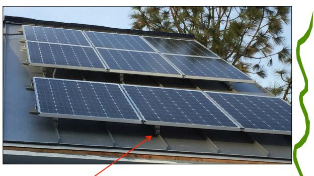
S-5! clamps Firmly attach the roof, every 1.5-2' (not 3.5-4')
