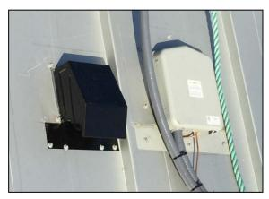
Working together: roofer flashes junction box like any other vent
