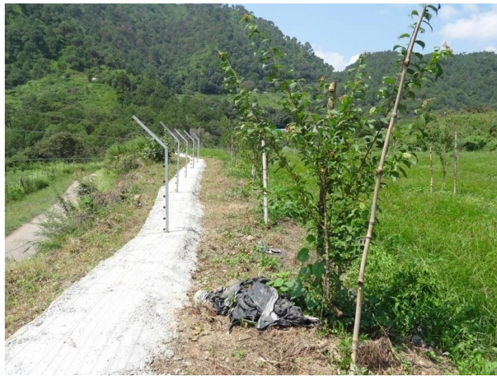
Pictures of solar fencing system established in Dr.YSPUHF, NaniSolan
