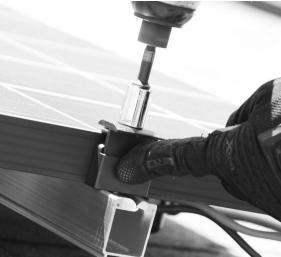
Do a final check to be sure that all installation hardware on the array is properly tightened to 12 ft-lbs.
