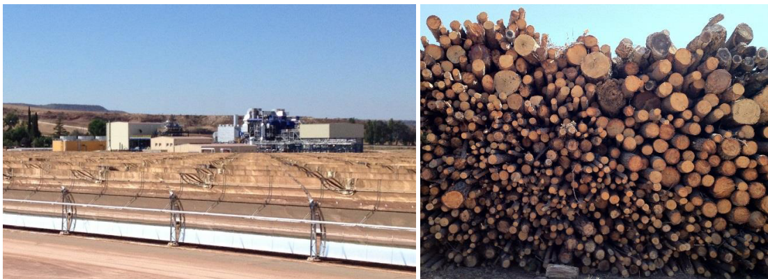
Figure 1: First CSP-biomass plant under construction near Lleida, Spain (left) and biomass fuel (right)
