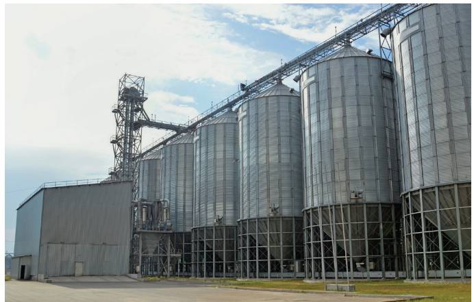
Figure 3: Silos used to store malt and barley
