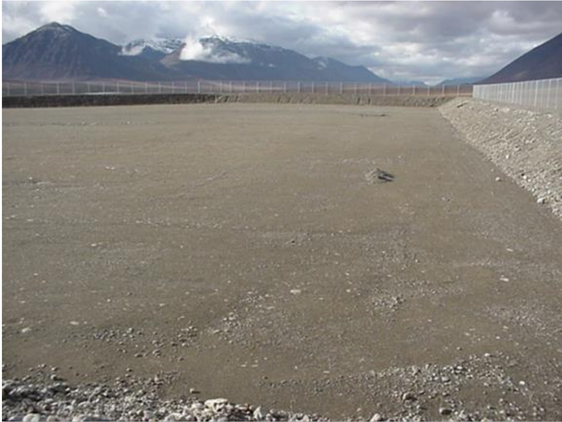
An example of a landfill built on a pad above permafrost prior to waste placement
