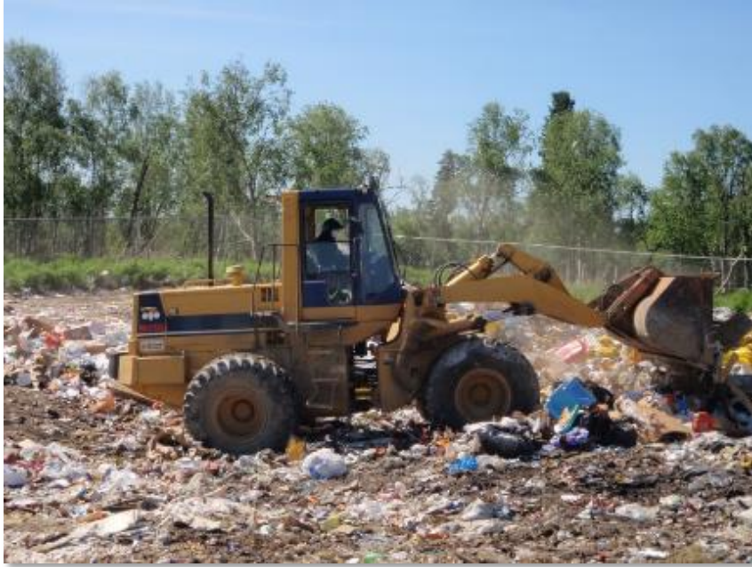
Landfill operator consolidating and compacting waste.
