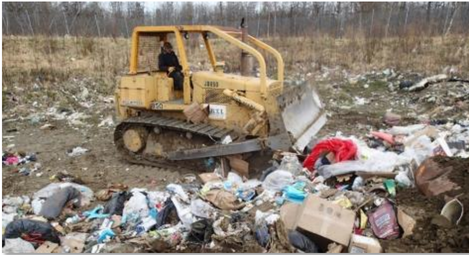
Operator using a dozer to consolidate waste.
