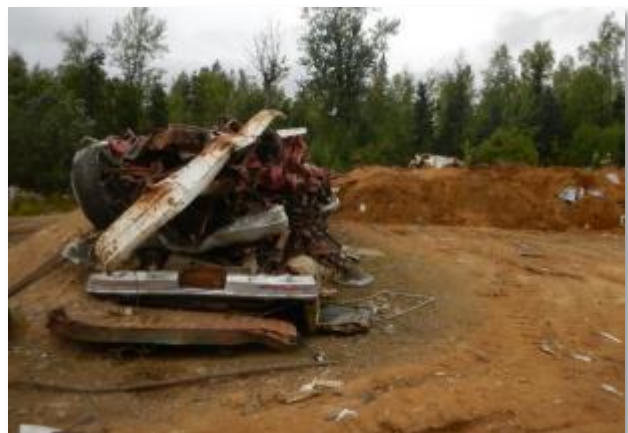
Vehicles used as a berm to mark the edge of the working face.
