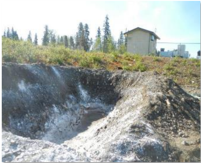
Septage trench with lime added.
