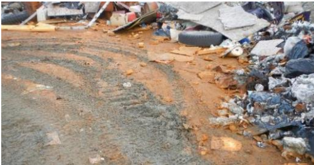
Orange staining near the waste caused by leachate. The waste should be covered to prevent the formation of leachate.
