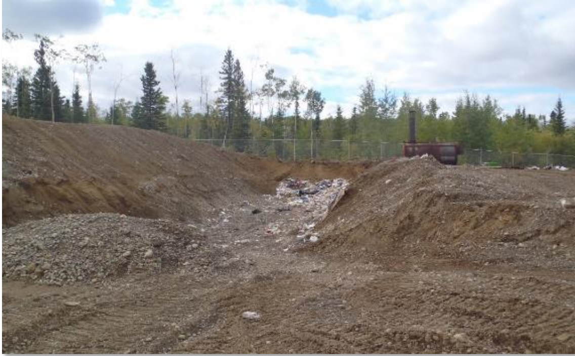
Trench-and-fill working face.
