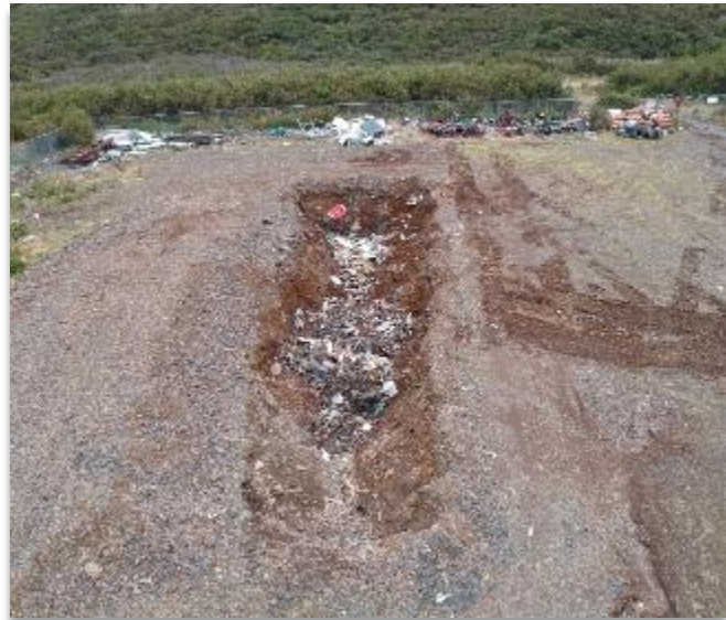
Trench-and-Fill landfill. All the waste is consolidated into one half of the trench. Notice that the waste is not spread across the site.
