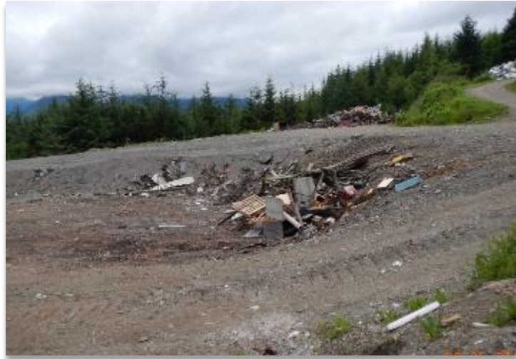
Working face at an area fill.
