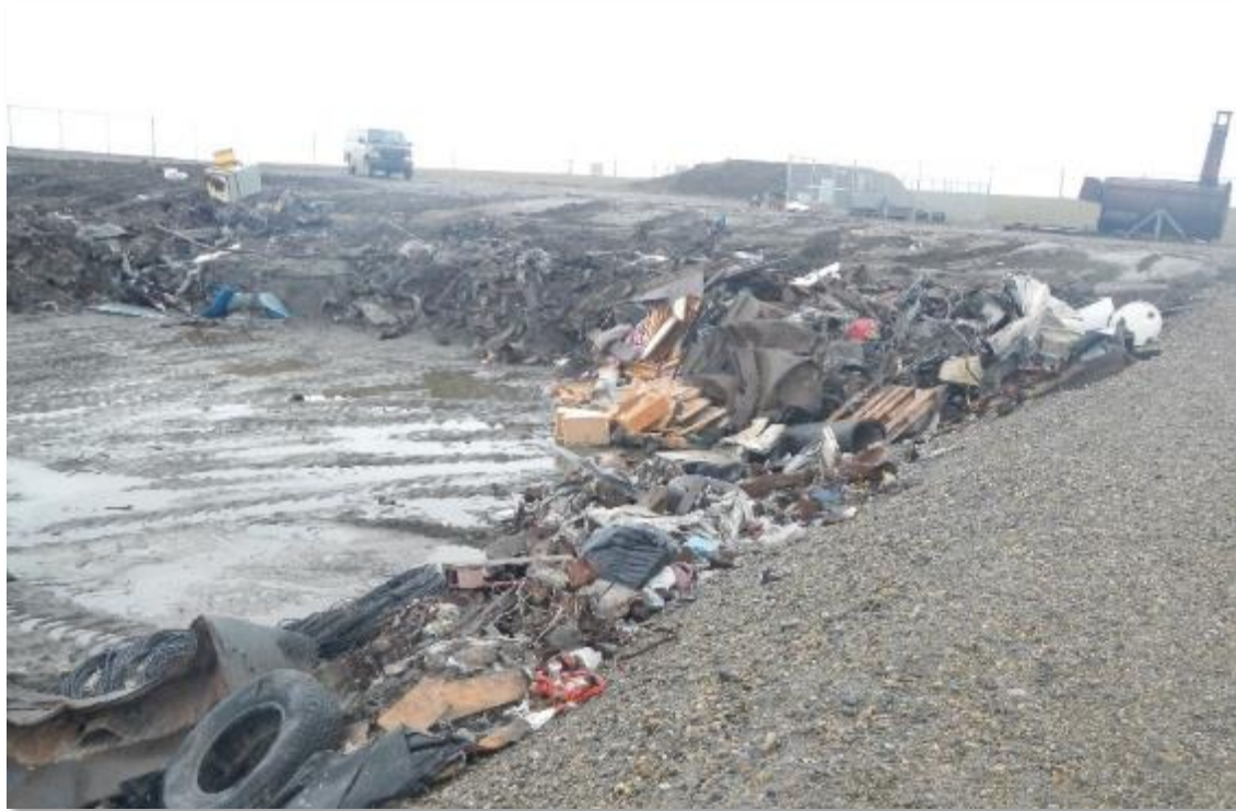
Working face at an area fill landfill.
