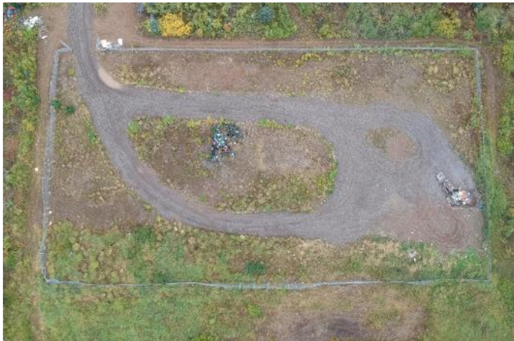
Well-maintained road within the landfill.
