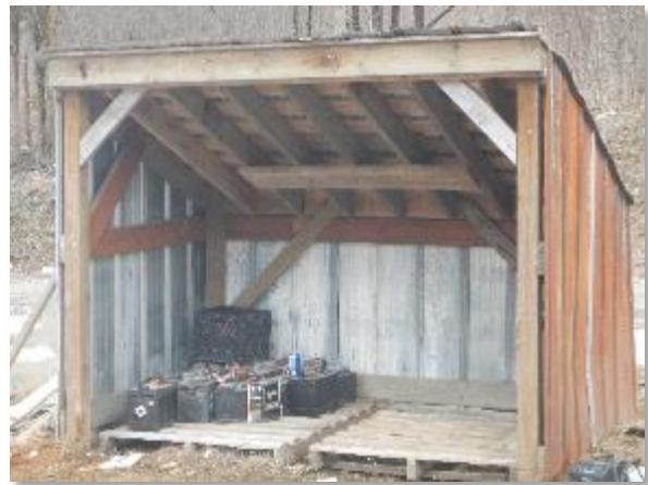
Covered storage shed for lead acid batteries.
