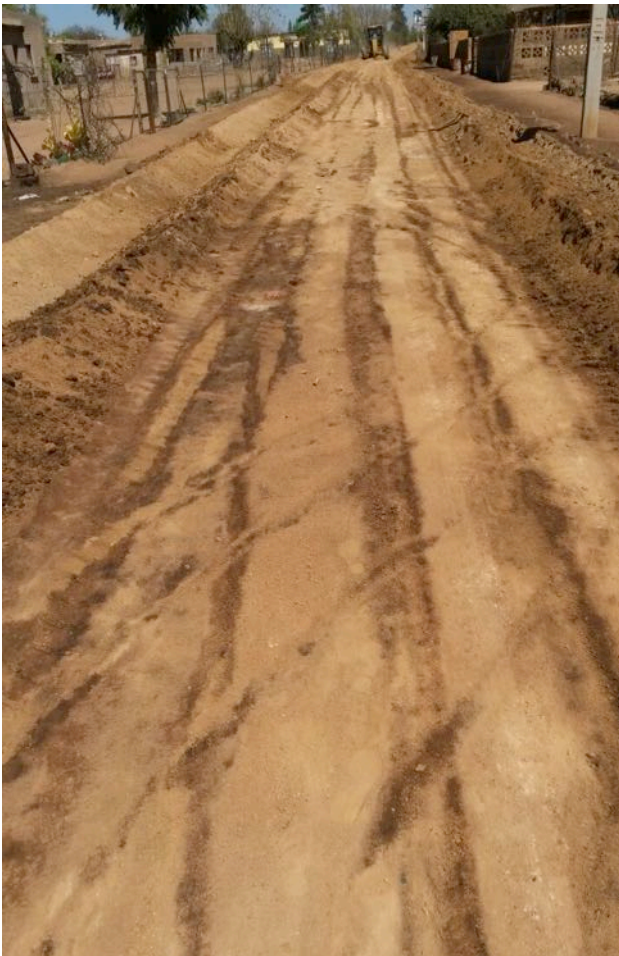
(1) Surface of road is scarified.
