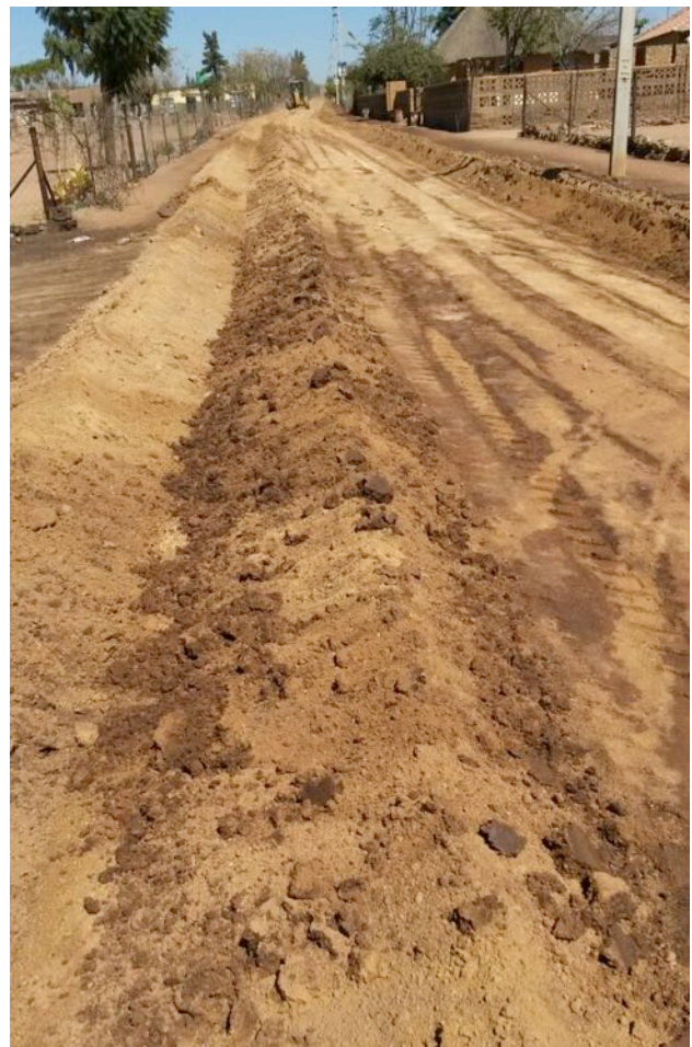
(2) Windrows are created and for the GreenBit product to be mixed in.
