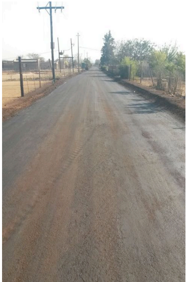
(8) The surface of the road is sealed.
