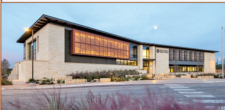
Bexar County's Public Works Department's office building. Photo from Marmon Mok LLP.
