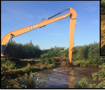
SAB Field Supervisor Tony Meade and Field Technician Luke Chaisson installing a silt boom to catch any disturbed sediment travelling downstream during excavation.
