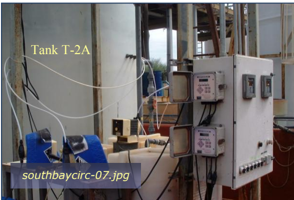
Photo #5: IWTP ORP and pH Metering Taken By: Greg V. Arthur Date: 08/11/09
