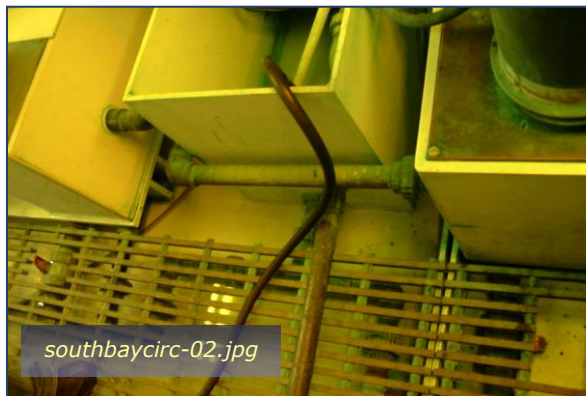
Photo #7: Secondary Containment Pans/Trenches Taken By: Greg V. Arthur Date: 08/11/09
