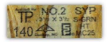
Properties are determined by either mechanical grading (testing) or visual grading. Most is visually
