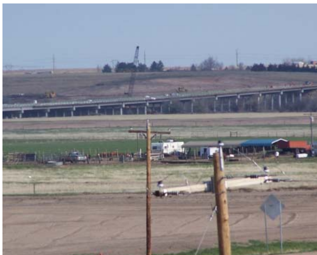
Figure 3. Looking southeast from US-50 at the New Arkansas River bridge.
