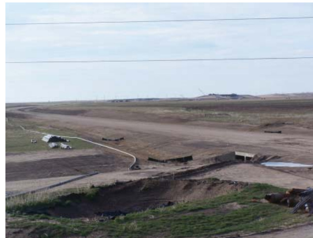
Figure 2. Roadway and drainage construction south of Marshall Road.
