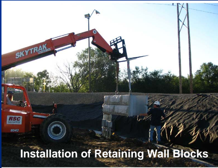
Installation of Retaining Wall Blocks
