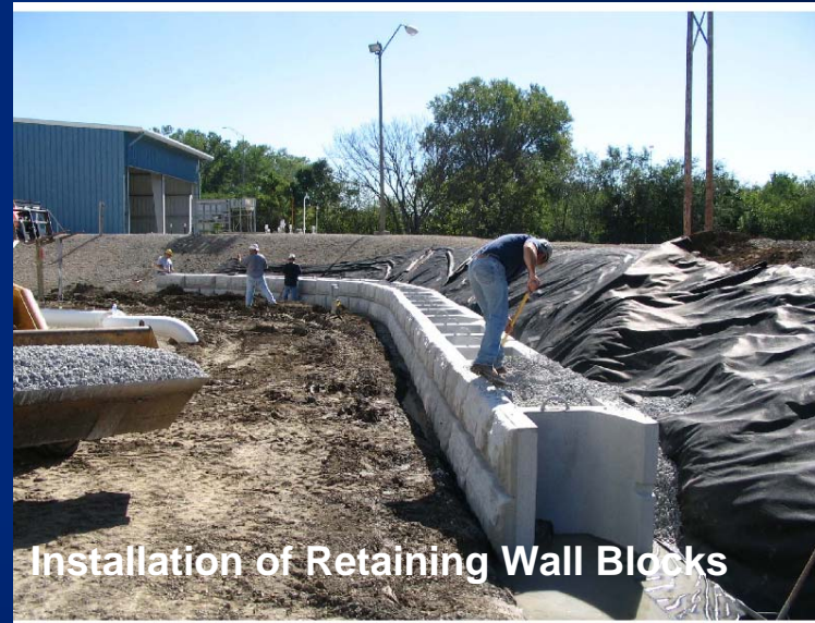
Installation of Retaining Wall Blocks
