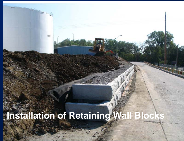
Installation of Retaining Wall Blocks
