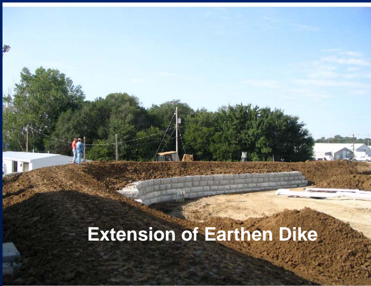
Installation of Retaining Wall Blocks
