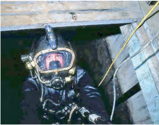
Gissendanner, UT grad, 110 ft water reservoir gates inspection.
